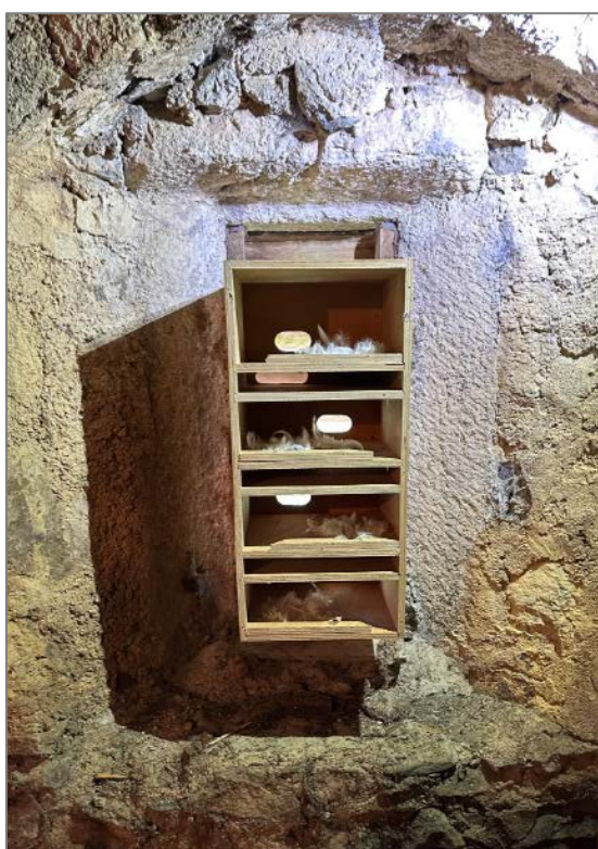
Fig. 3: Example of 2 separate colony boxes (with back section removed for illustration) installed with the remaining louvre meshed to restrict access into the bell tower.
