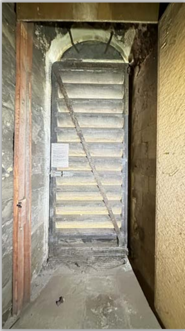
Fig 1. Current internal louvre design.
