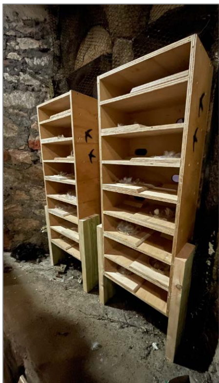
Fig. 3: Example of 2 separate colony boxes (with back section removed for illustration) installed with the remaining louvre meshed to restrict access into the bell tower.
